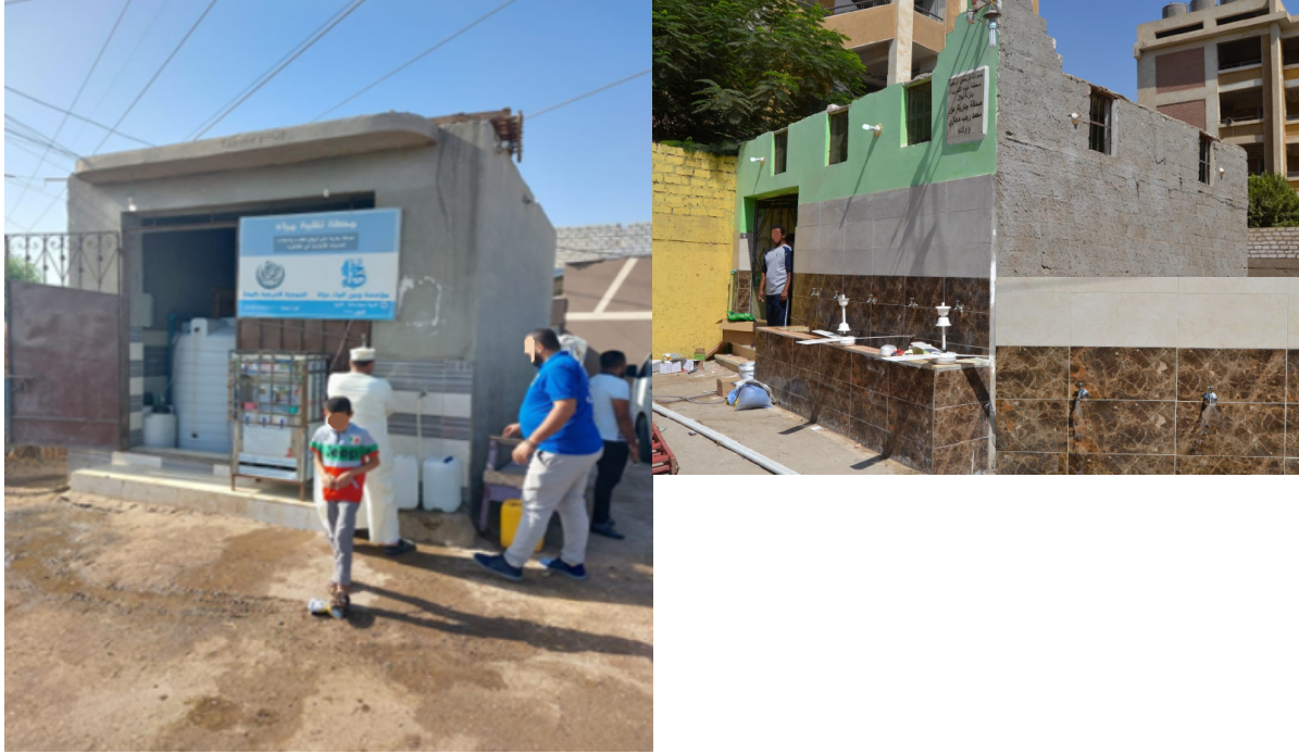
Figure B1. Water Treatment Units
